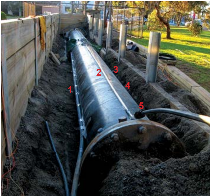
Opposite view during sensor installation
